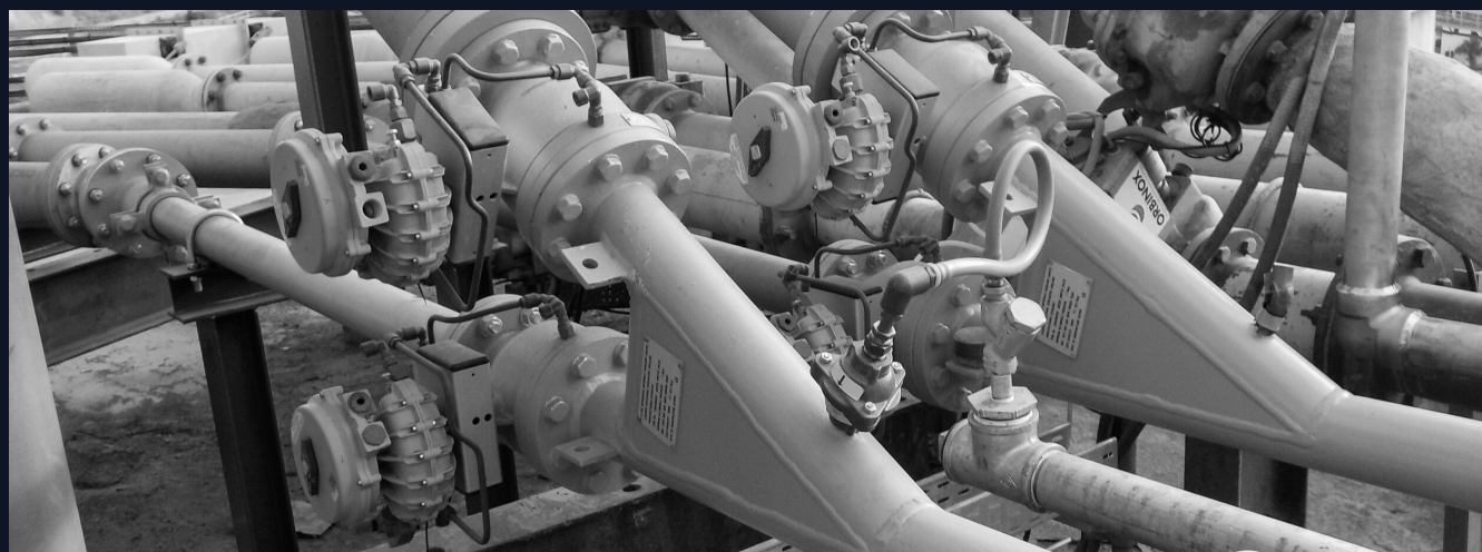
A pair of inline Dome Valves used to divert material in a pneumatic conveying pipeline, also known as a Dome type Switching Valve
